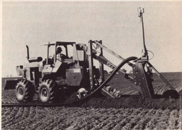
Agricultural drainage installation package consists of the R100 trencher fitted with a 'Tiling' boot also designed and built by Ditch Witch.
